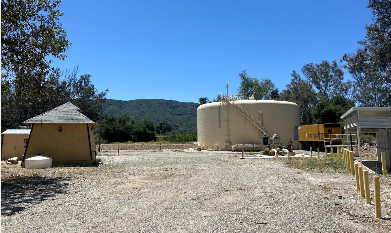
Photograph 19. View of existing tank at OWS Wellfield laydown yard (east of San Antonio Creek), facing south.
