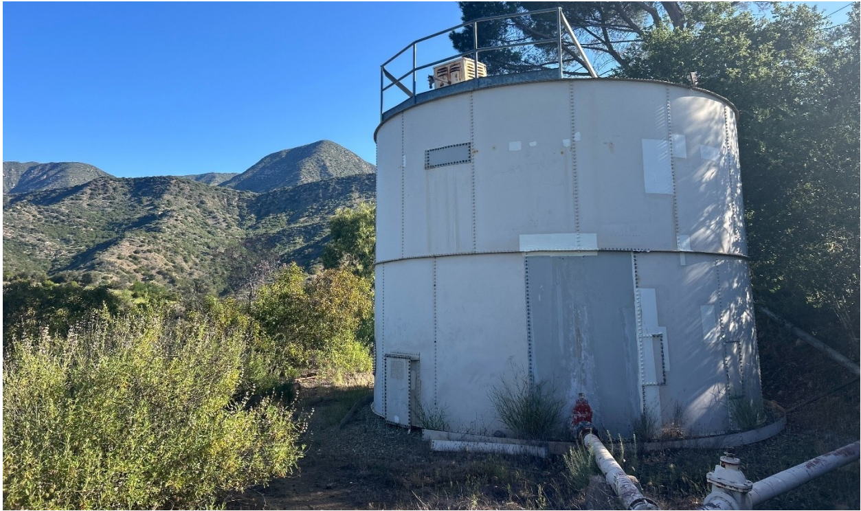
Photograph 1. View of existing tank at the Running Ridge Tank site with surrounding black sage – California sagebrush scrub vegetation, facing north.
