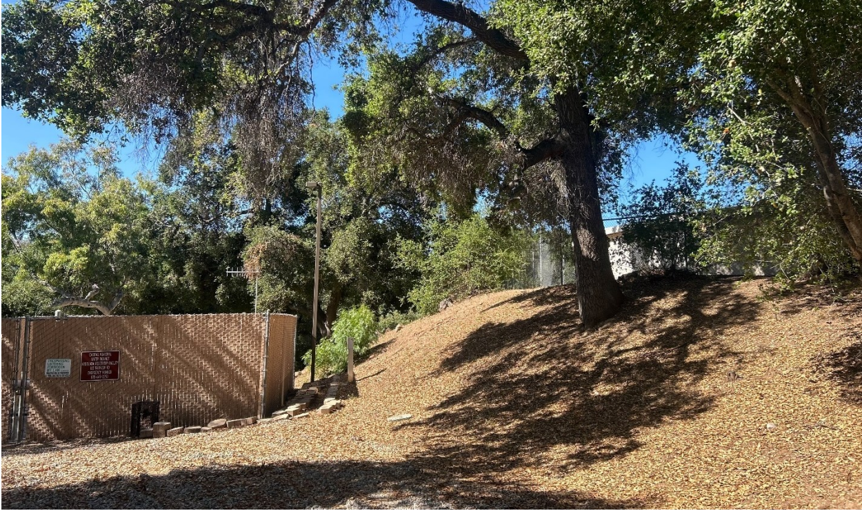
Photograph 5. View of existing Arbolada Tank and Pump Station site in the developed oak woodland, facing southwest.
