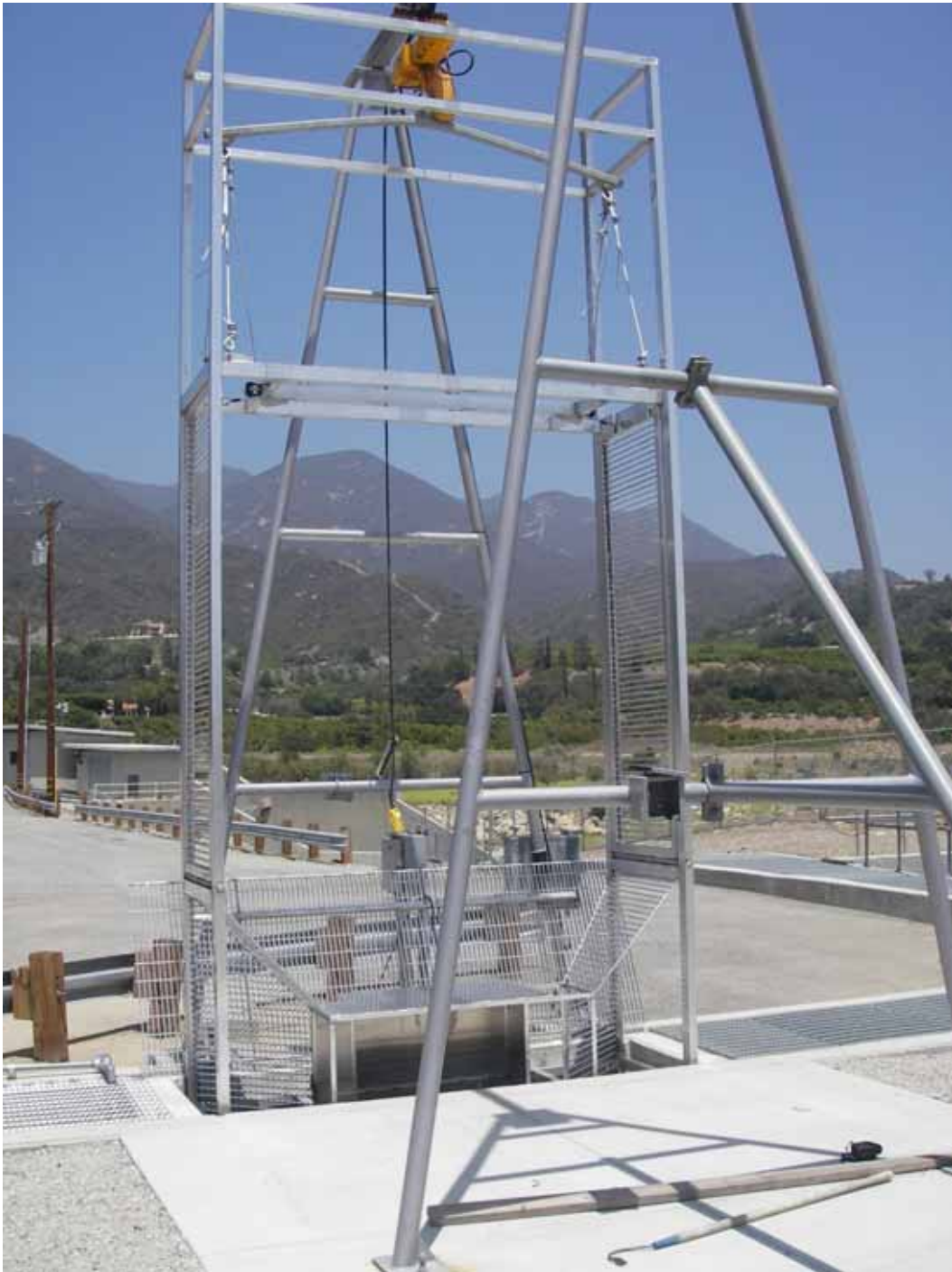
Appendix 5. Photo of the new fish crowder that directs migrants through the Vaki Riverwatcher scanner. The crowder is out of fish bypass and not operational in photo. Also in the photo is an A-frame and hoist that was completed and will allow for easy removal of the crowder for cleaning and repair.
